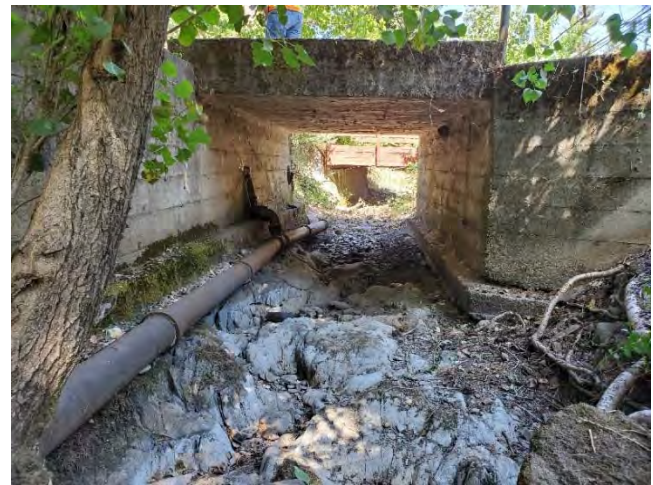
Sections 3 & 4 – Cedar Ravine Creek running in front of buildings and under driveway crossings with services laterals connected to the 6” CIP sewer main in the creek. Creek has rock bottom and trees.
